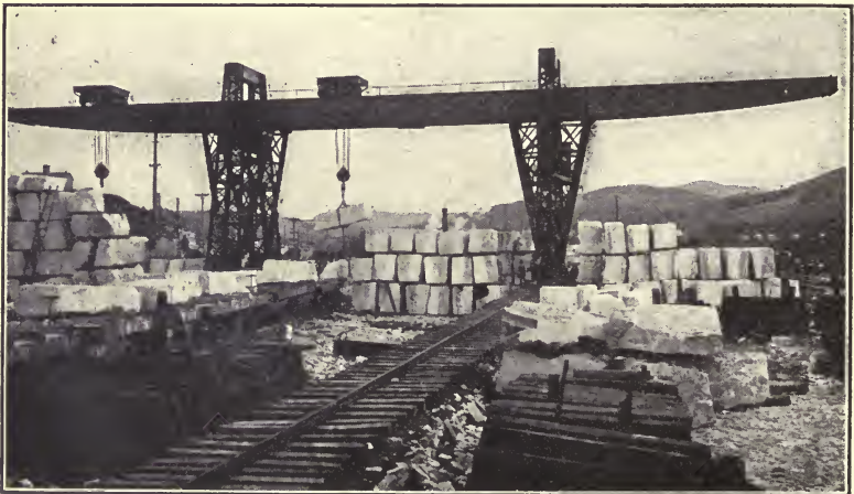
ELECTRICALLY-OPERATED GANTRY CRANE SERVING BLOCK FILE
